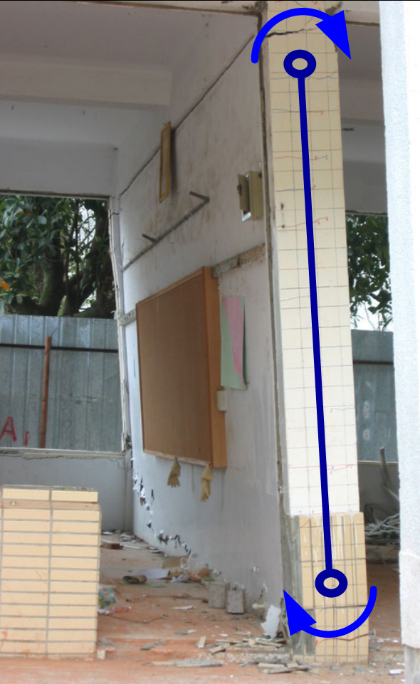
Frame 3 Brick Wall
