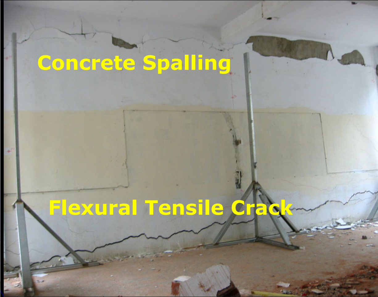
Frame 2 Brick Wall
